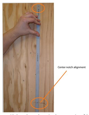
3 Use the provided template to determine the center points of the wall mounts. The "V" notches are labeled "L" for a landscape display or "P" for a portrait display. Use the appropriate "V" notch to align with the horizontal line drawn in the previous step.
